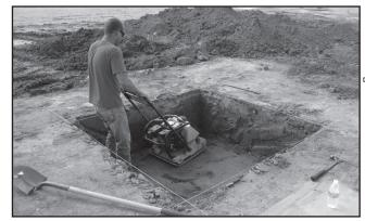
Soil Density compacted to 95% per ASTM-698
